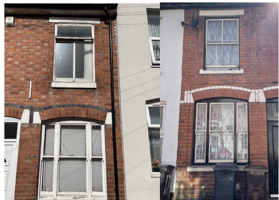
© Arup Figure 22: Some properties have original wooden windows
