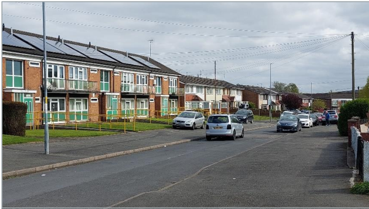
Housing along Coalway Road
