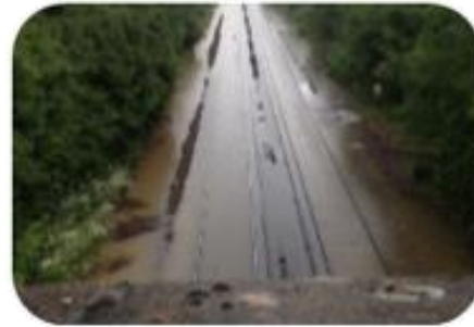
Rivers and heavy rain can flood the track
