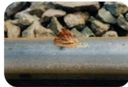
Leaves on the line make tracks slippery and affect connectivity
